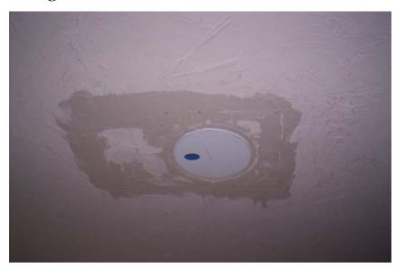
This area can now be sanded smooth. If properly done, you will never be aware of this joint, only the .010" seam round the cover plate which is minimal. Clean out the recessed cover groove, clean up the magnets and check for proper seating so the cover plate will be held in securely and flush. When finished attach safety cable with screws provided on the ring and panel.
